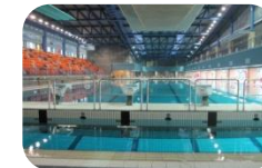
Movable bulkhead (Taiwan)
